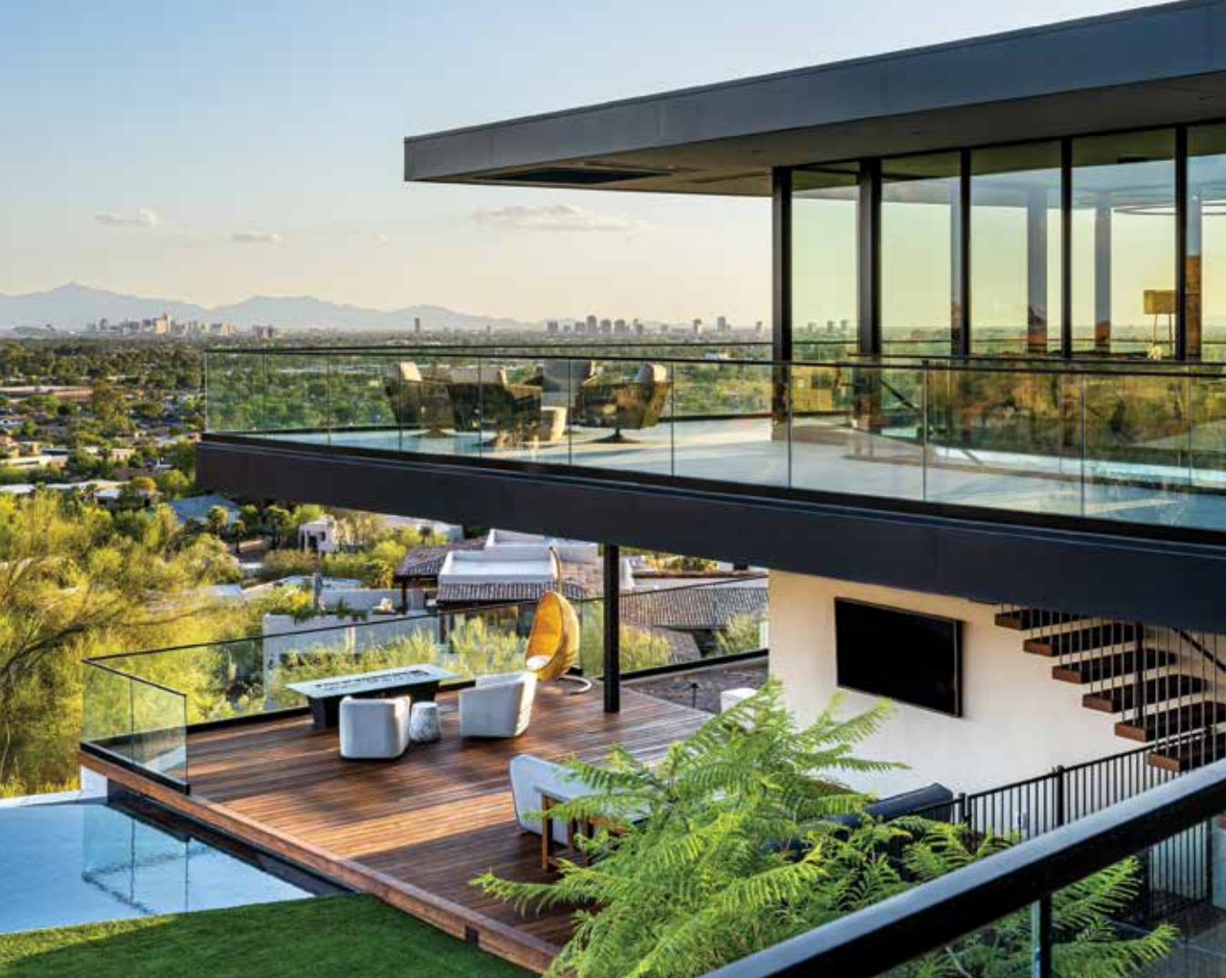
From top: The home contains guest rooms, a theater and the garage downstairs. The living room, dining room, kitchen and primary suite are on the upper level; in the theater, a sectional from Lee Industries—upholstered in Opuzen velvet—tops a patterned cowhide rug from Surya. The walls are upholstered in a wool fabric from Brentano. The throw pillows are made with fabric from Jim Thompson. Opposite page: Architect Erik Peterson had very specific ideas for the home's three stairwells, including the one at right, which was partially inspired by Frank Lloyd Wright's Fallingwater.
